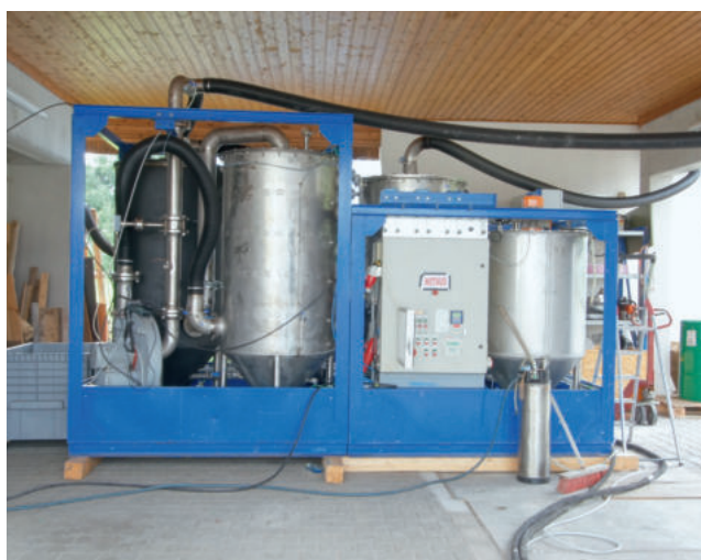
Figure 5: Carrying out tests at Bad Orb
