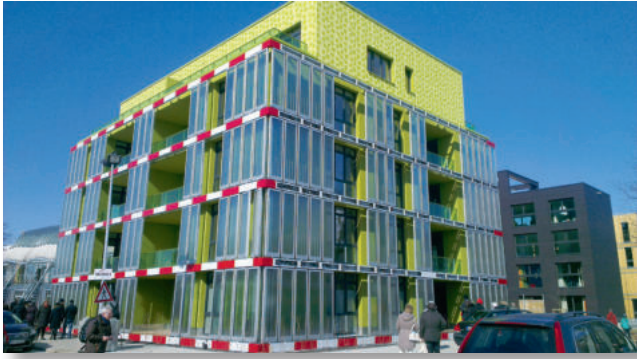
Figure 7: Prototype for the use of algae for domestic supply of power and heat in the Wilhelmsburg district of Hamburg (source: Martin Kerner/SCC)
